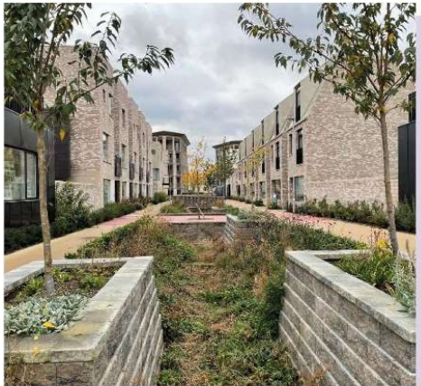
A car-free link route can incorporate food growing and sustainable drainage systems
